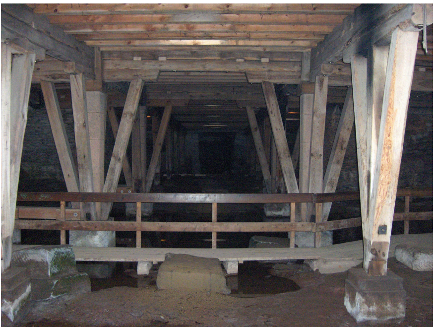
Wooden pillars supporting the arena floor, Trier
